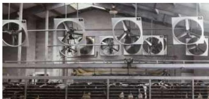
FIG. 9. Circulation fans and sprinklers over holding area.
